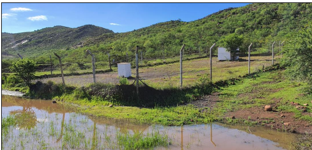
Figure 15: General view of the magazine housing the explosives
