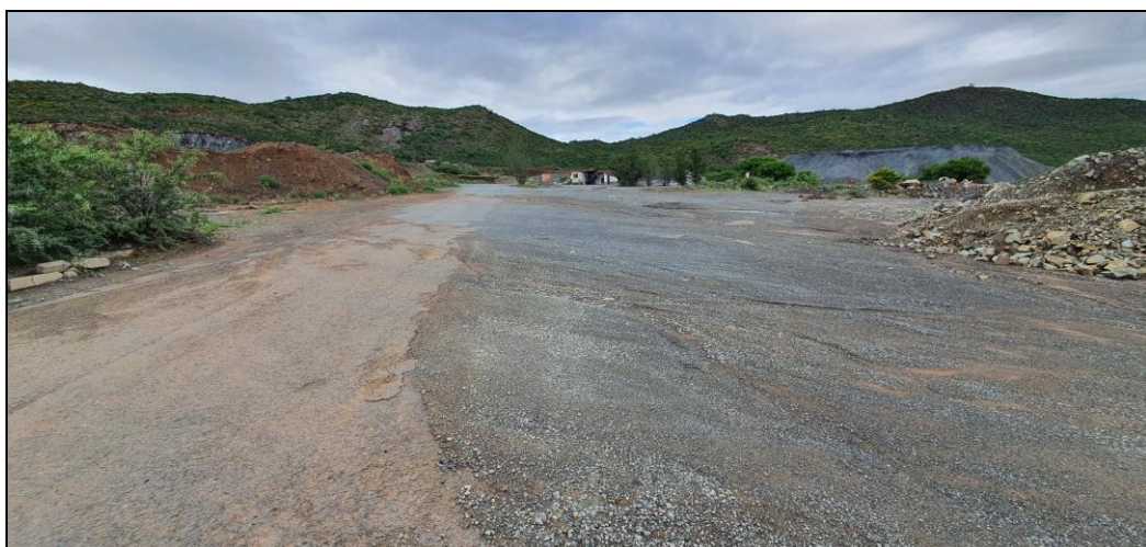
Figure 9: General view of one of the access roads to the quarry
