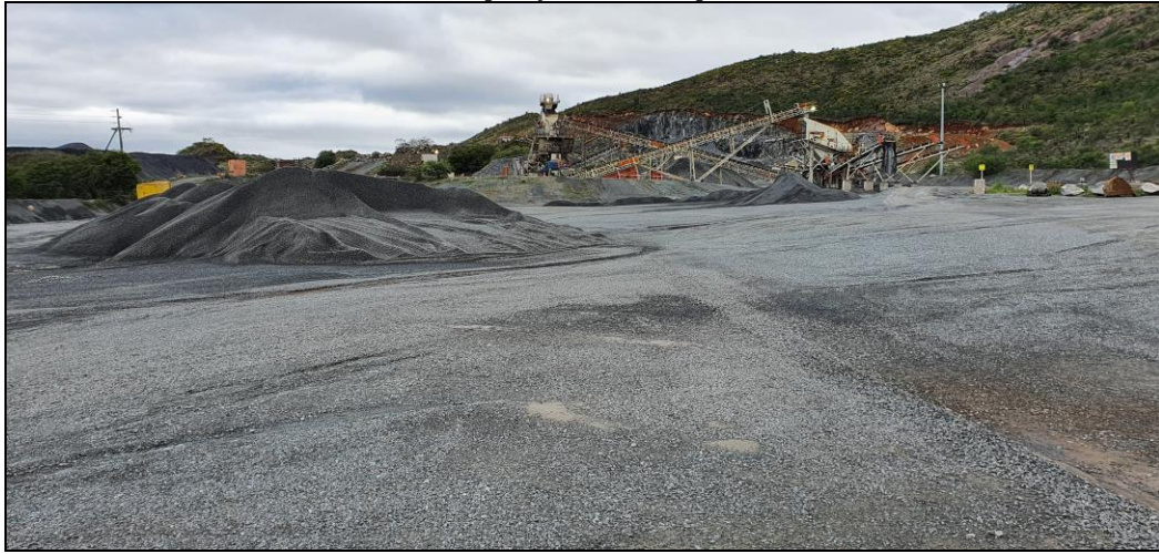
Figure 10: General view of the processing area and central section of the mine
