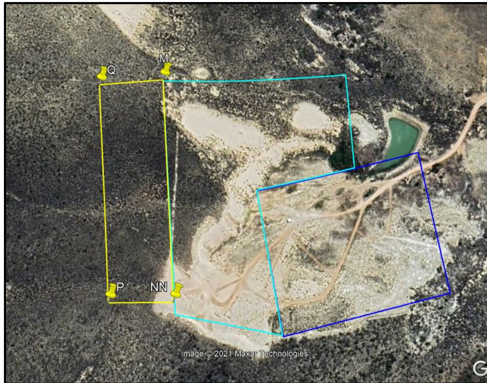
Figure 2: Satellite view showing the position of Site Alternative 3 (EIA preferred alternative) within the surrounding landscape, where the blue polygons show the current mining footprint, and the yellow polygon shows the proposed extension area (S3). (Image obtained from Google Earth).
