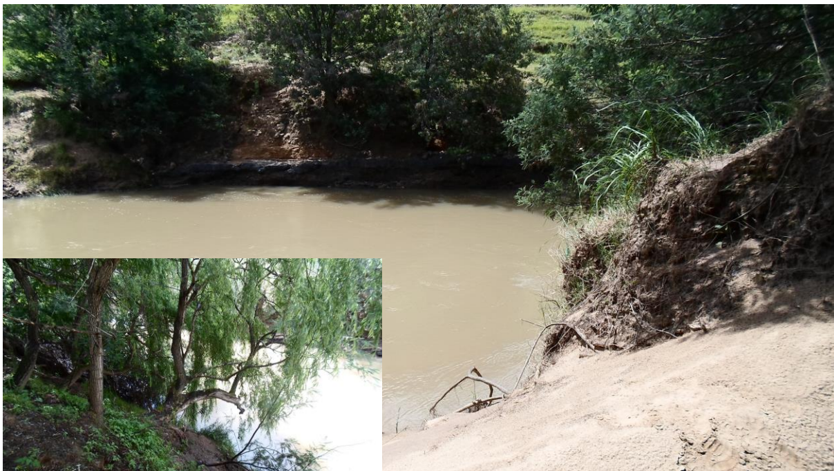
Figure 14: Photograph of the alien vegetation ( Acacia dealbata and Salix babylonica ) on the embankments of the Tsitsa River (November, 2022)
