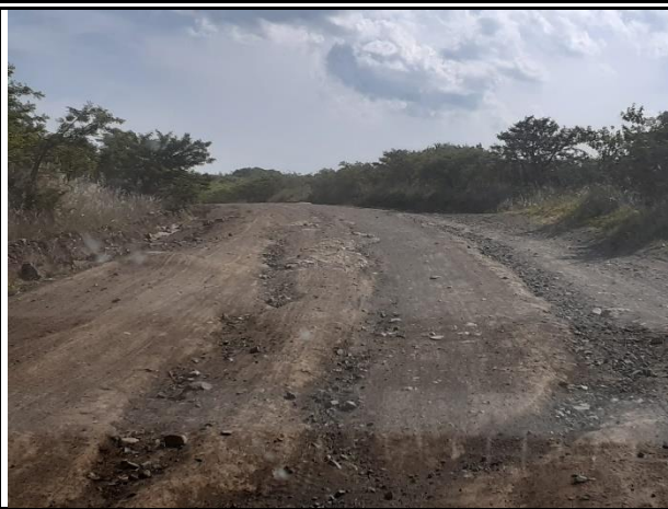
Erosion – road must be repaired
