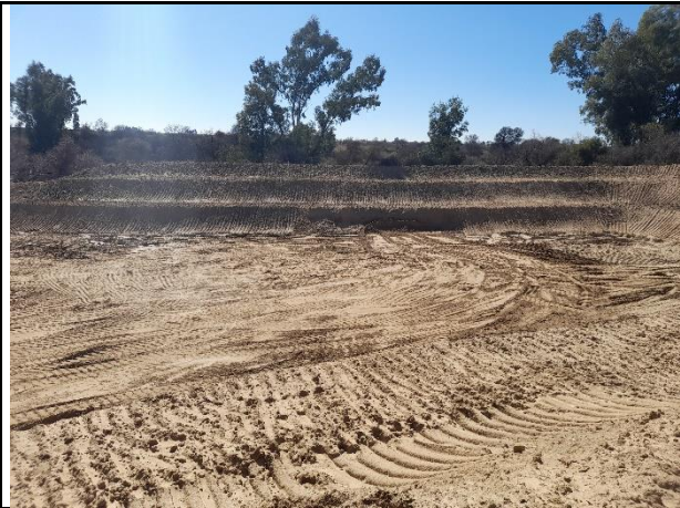
Neatly sloped mining benches
