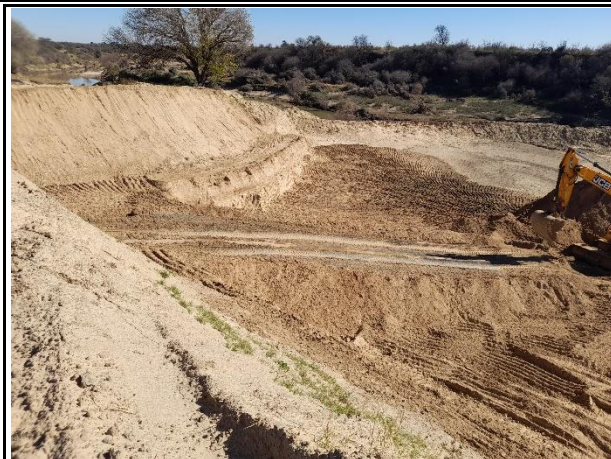
Rehabilitation of mining area in progress
