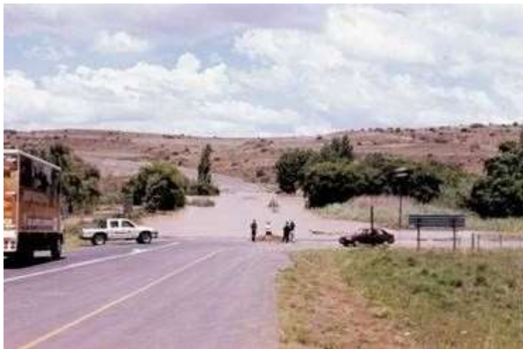
Figure 5: Flooding of the R26 prior to the raising of the Jim Fouché bridge (image obtained from https://www.hydropower.org/case-studies/south-africa-welbedacht )
