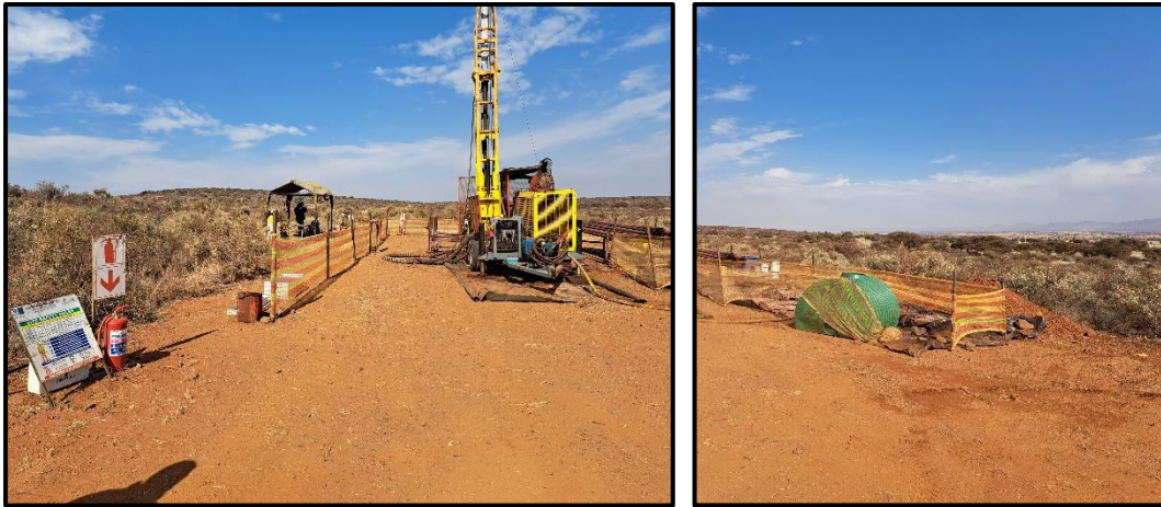
Figure 2: Example of a typical drill site.
