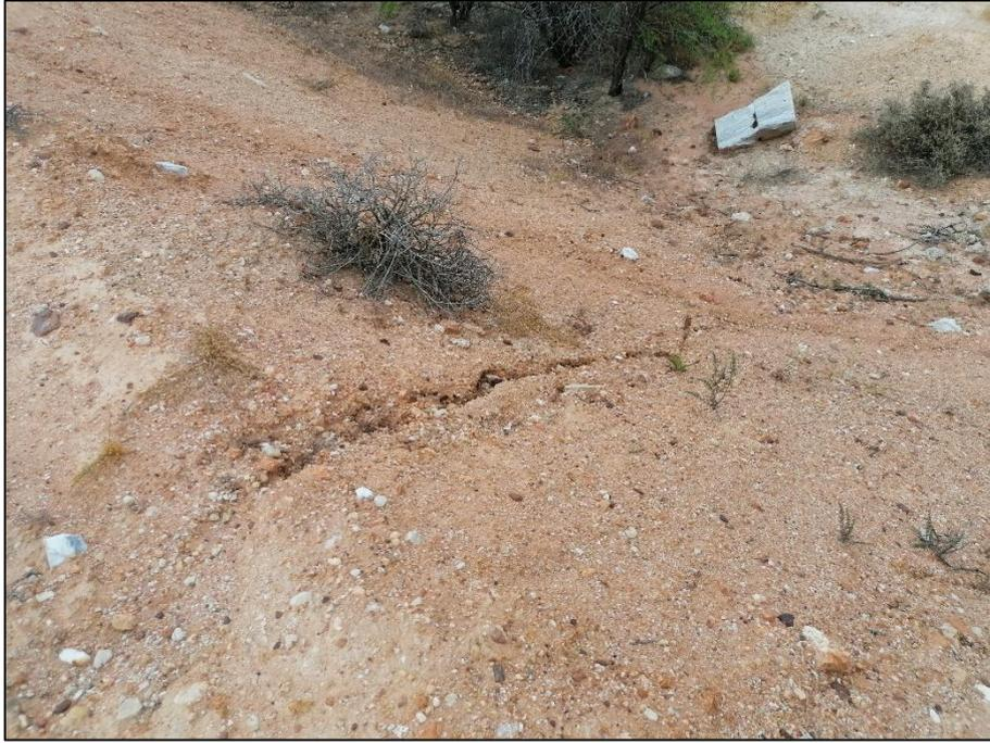
*Figure 36 Soil capping and erosion on the berm around the old mine*
