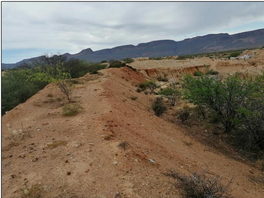
*Figure 37 Soil capping and erosion on the berm around the old mine*
