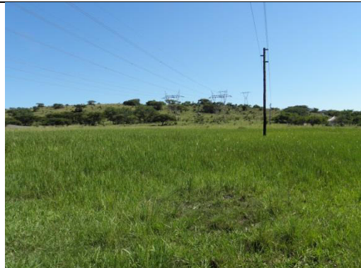
Photo 12: Power line traversing the HS (Pylon placed within the seasonally saturated zone).
