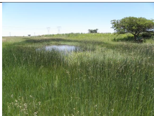
Photo 6: Artificial depression within VB created downstream of the culvert (seasonally saturated)
