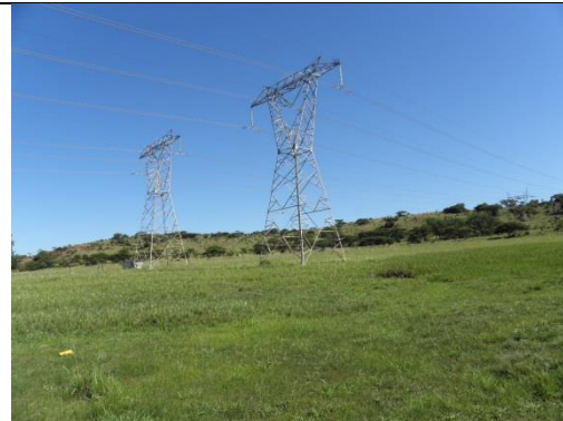
Photo 13 Transition area between the seasonally saturated zone (top left corner of wetland area) and temporary zone (rest of wetland area). Note the power lines traversing the HS.
