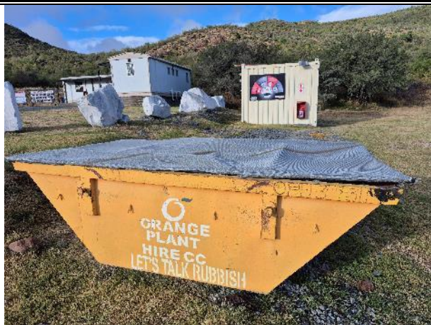
Cover placed on skip to prevent scavenging
