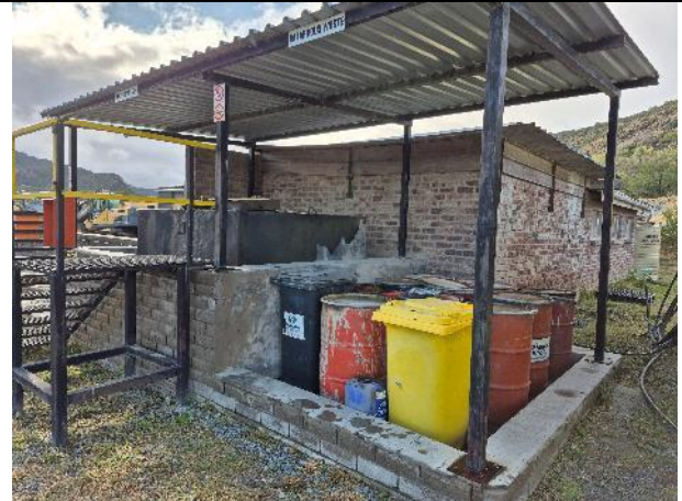
Bund of used oil storage area to be sealed
