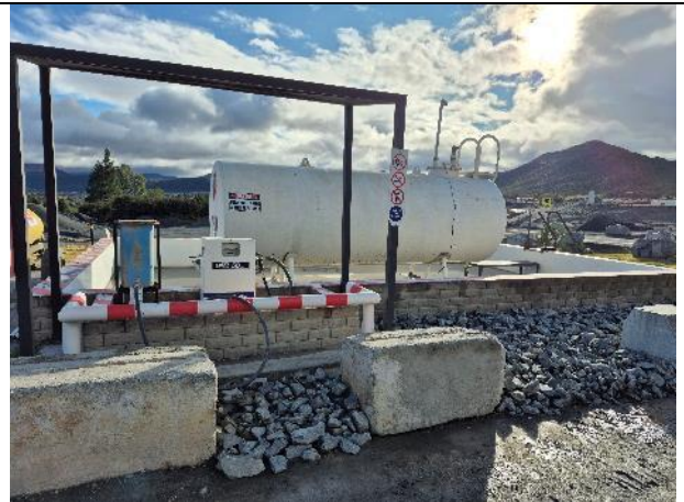
Bund of diesel tank to be sealed
