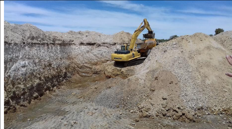
Example of how the excavation area
