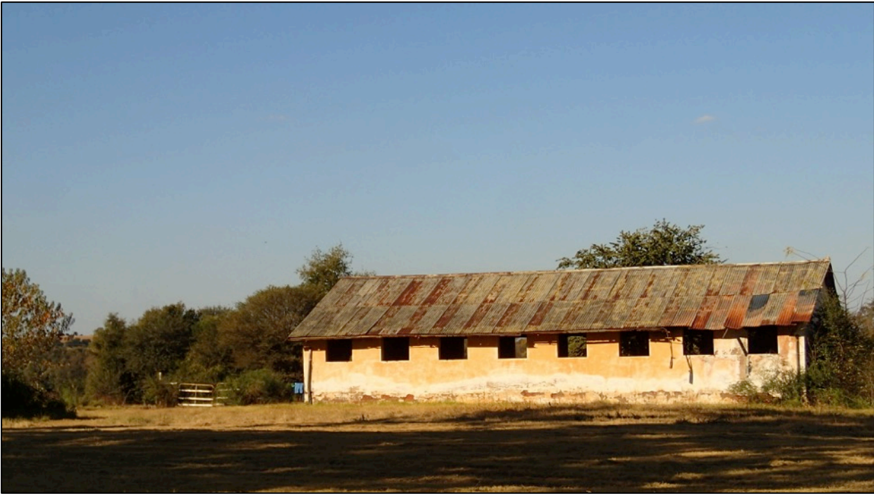
Figure 16. The "Barn" structure at Site 002
