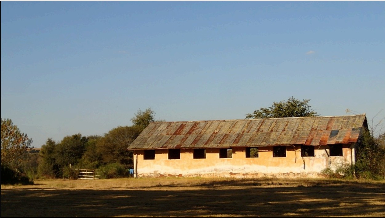
Figure 16. The "Barn" structure at Site 002
