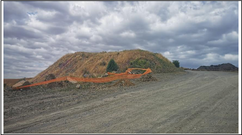
BERMS SURROUNDING CONSTRUCTION AREA
