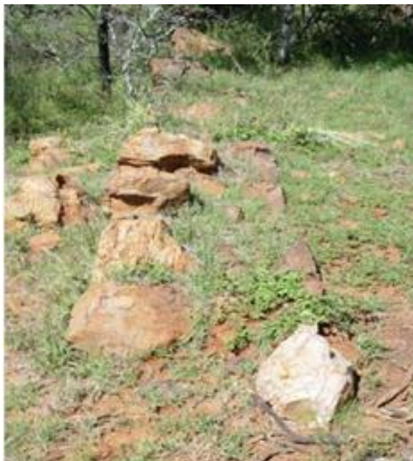
Figure 54: Section of the square foundation (Image obtained from Pure Source Mine Final Scoping Report done by Shango Solutions)
