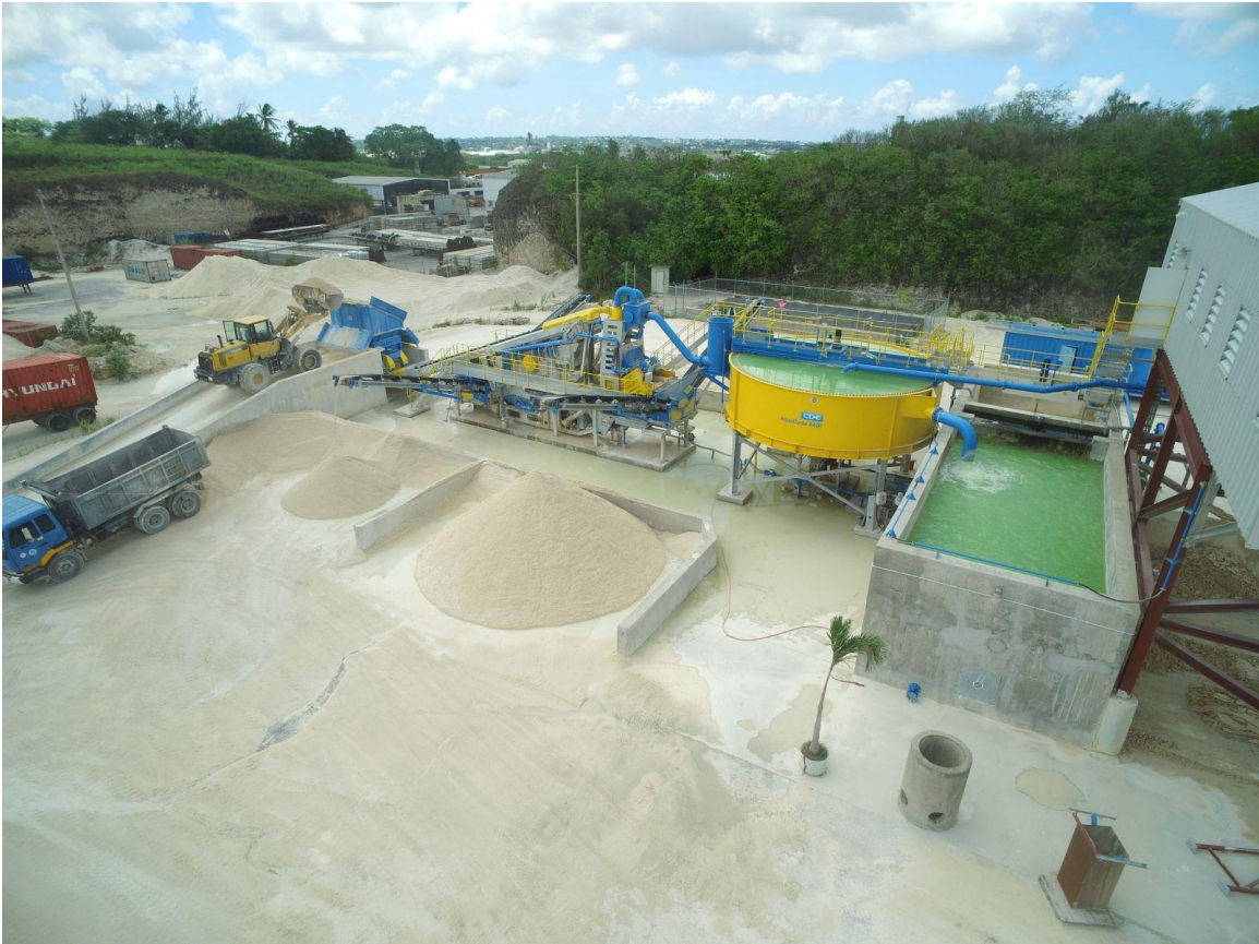
Figure 17: Example of a EvoWash plant with AquaCycle(4)
