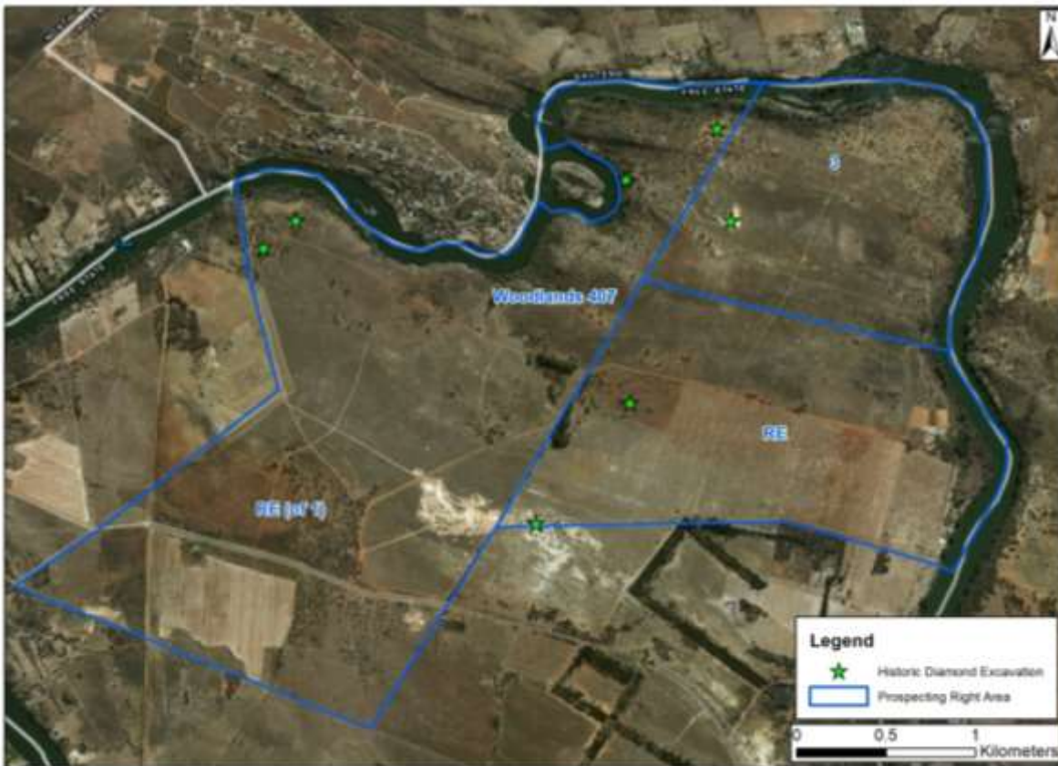
Figure 36: Encountered historic diggings (diamond excavations) during field investigations.
