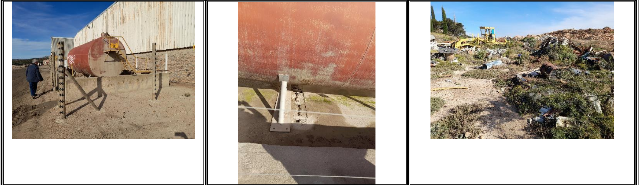
Bunded area to be sealed
