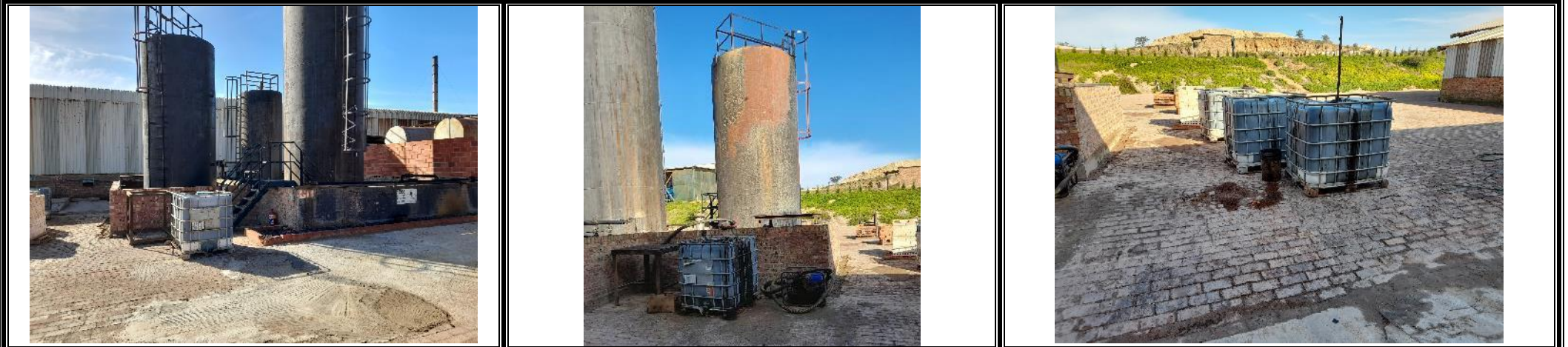
Used oil to be placed inside bunded areas
