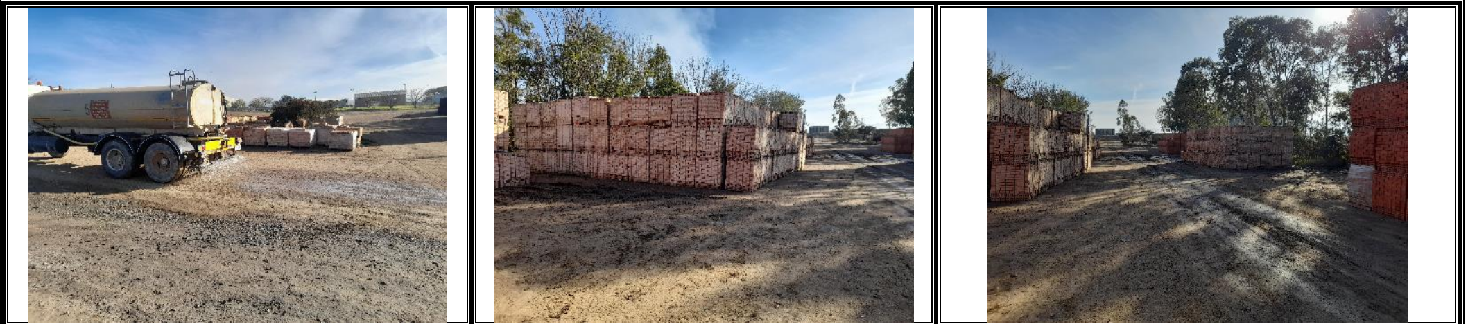
Dust suppression in progress
