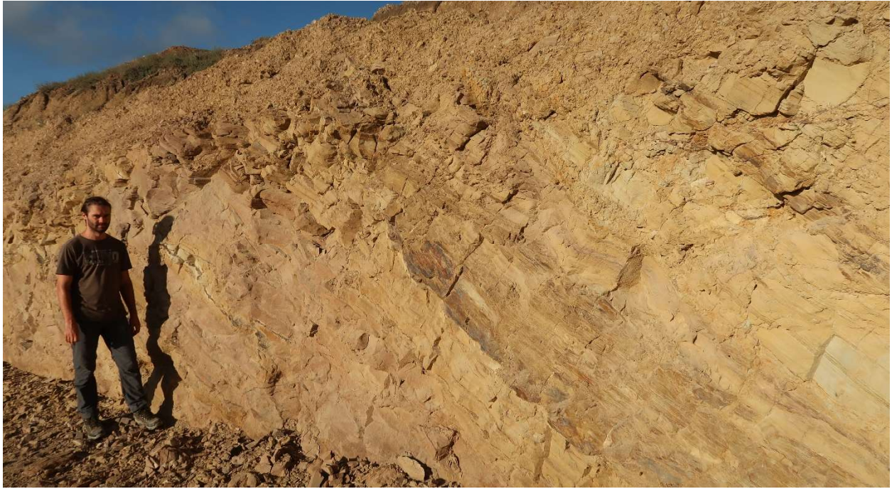
Figure 24: Moderately altered strata of the Waaipoort Formation exposed by deep excavations in the main brick clay quarry at point 10 (Fig.1).
