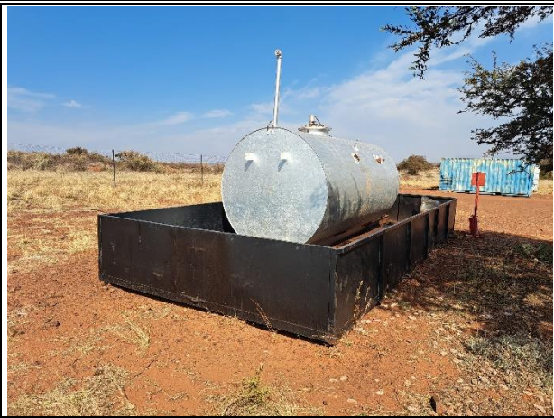
Well build drip tray installed around the diesel tank
