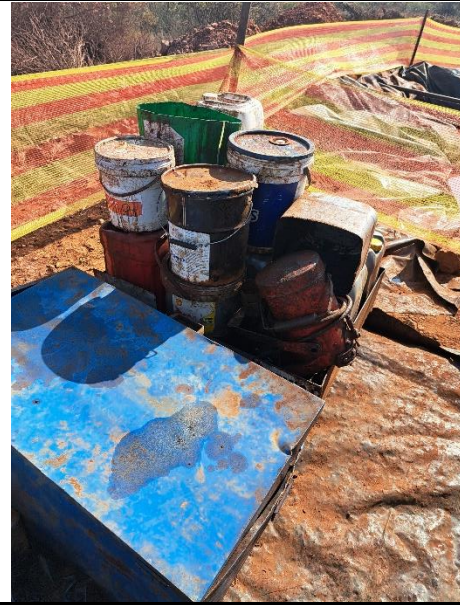
Operational site neatly managed
