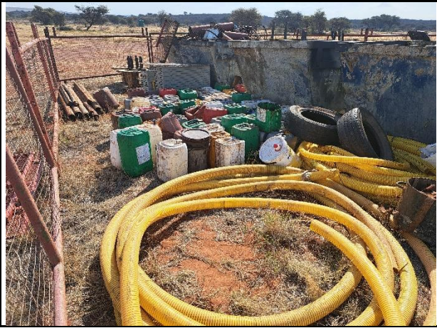
All chemicals must be kept in a bunded area with impermeable surface
