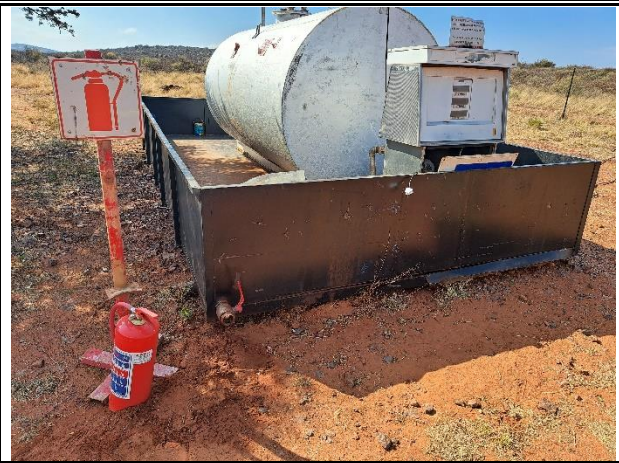
Well build drip tray installed around the diesel tank
