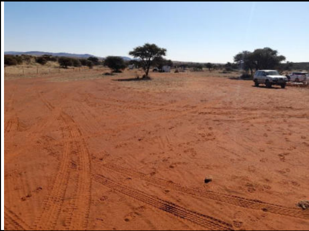
Neatly managed site camp
