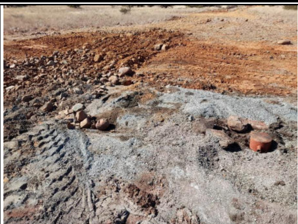
Capped drill site where hydrocarbon spills must be cleaned and rehabilitation still needs to be finalised
