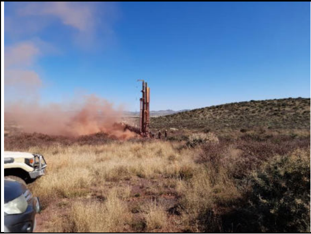
Drilling in progress
