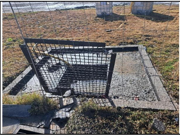
Wash bay with oil sump. Flow bins are visible in the back.
