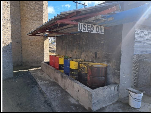
Used oil storage
