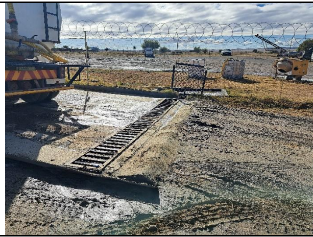
Wash bay with oil sump. Flow bins are visible in the back.
