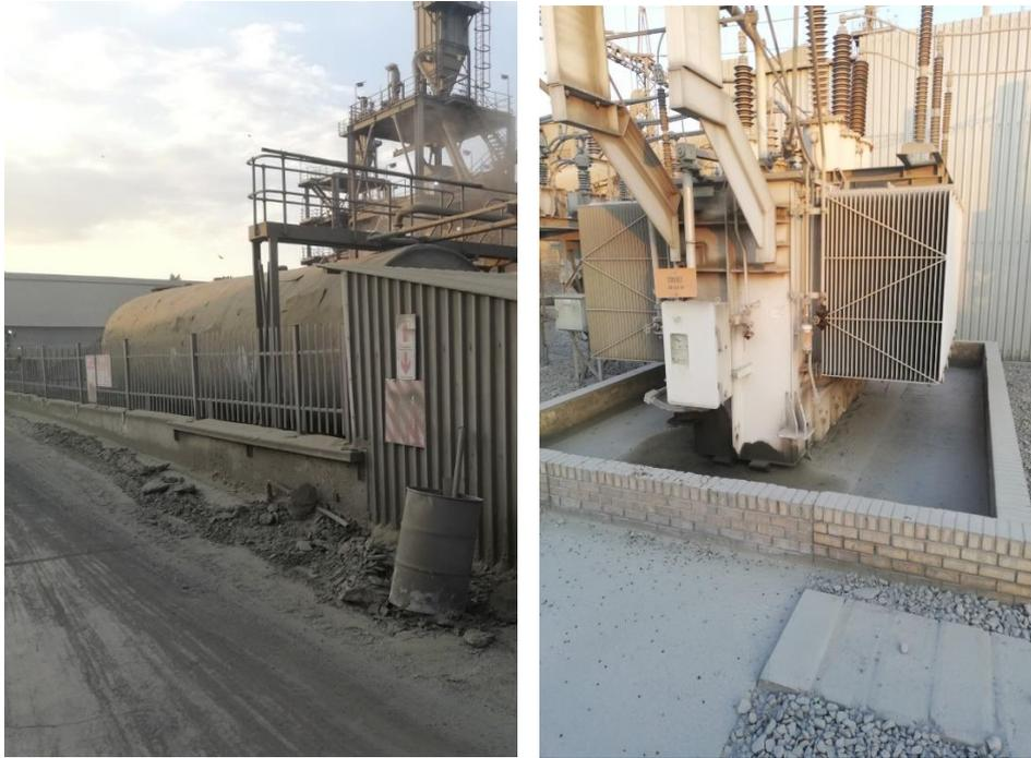
*Plate 4-5 Illustration of Bunded Fuel Tank and Bunded Sub-Station Areas*
