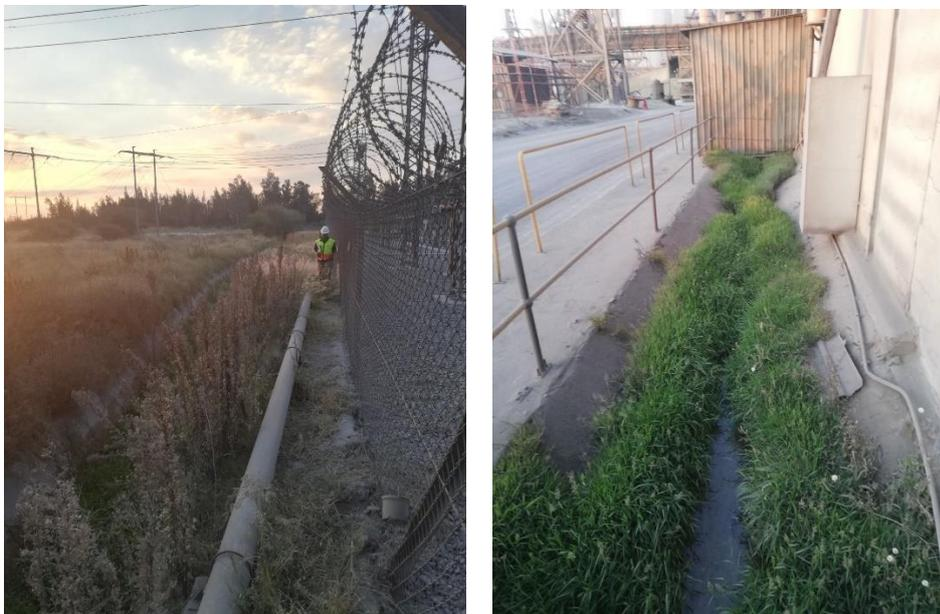
*Plate 4-6 Examples of Poorly Maintained Stormwater Channels*
