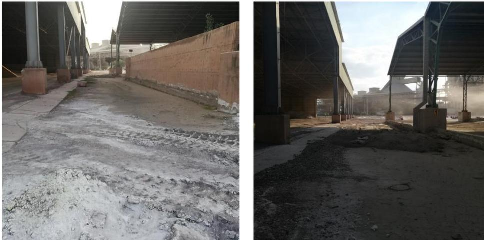
*Plate 4-8 Illustration of Blocked Channels in the Additives Storage Areas*
