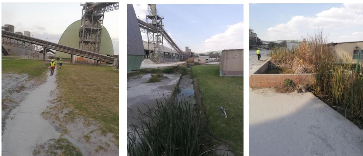
*Plate 4-7 Illustration of Poorly Maintained and Blocked Stormwater Channels in the China Town Area*
