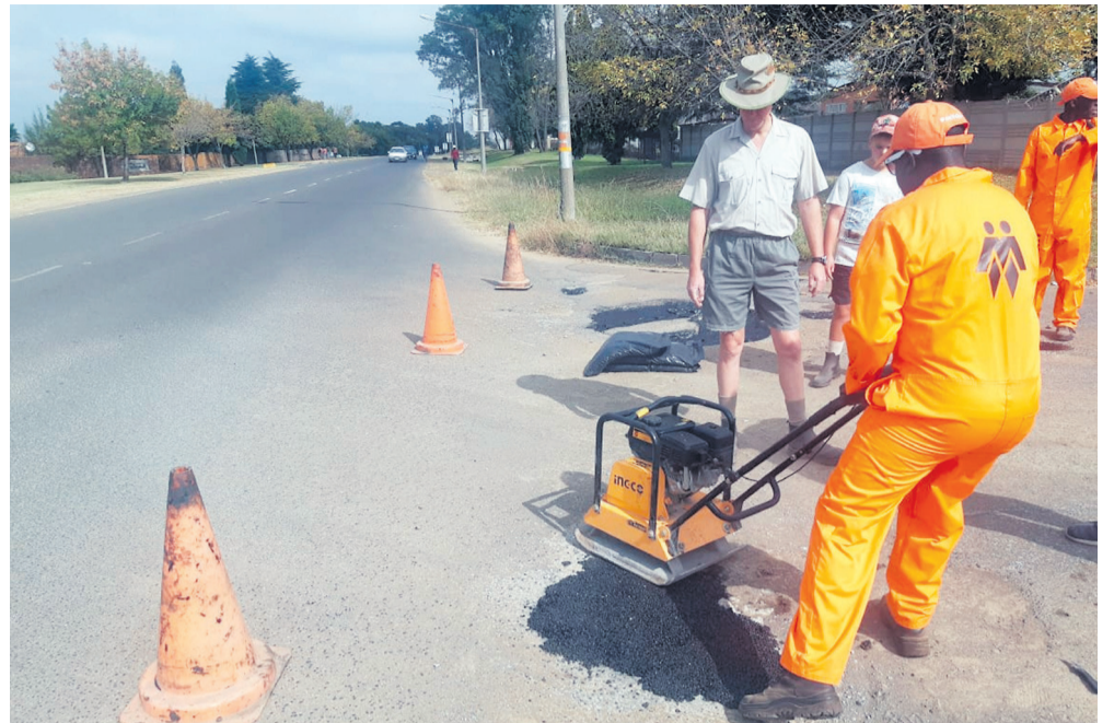
Resident from Buffel Street Mr Riaan Smit, looks on to see how AfriForum's Mr Xolani Mnisi closes up potholes in the street. (Photo: Supplied)
