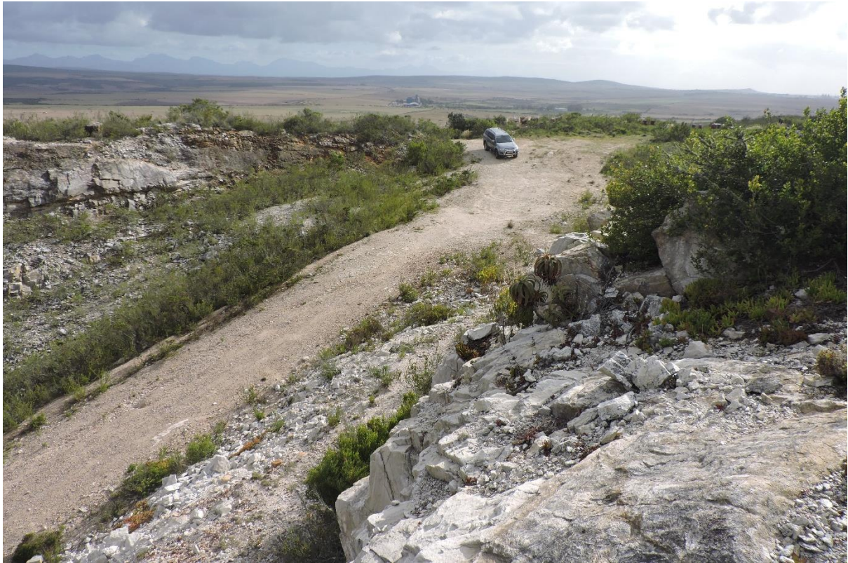
Figure A3: Part of the access road into the quarry
