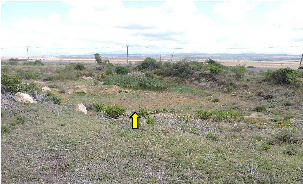
Figure A5: The arrow indicates a small earth-walled dam close to the N2
