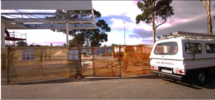
WALK IN ENTRANCE GATE TO CONSTRUCTION AREA
