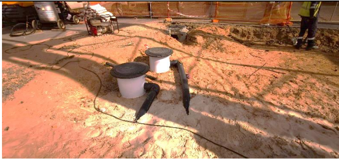
TWO FILLER PODS – FUEL TRUCKS WILL CONNECT DIRECTLY TO FILLER PODS TO REFILL STORAGE TANKS
