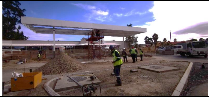
STORAGE TANKS INSTALLED AND TESTED, COMPACTED WITH RIVER SAND AND FITTED WITH TWO MANHOLES AND FOUR MONITORING HOLES
