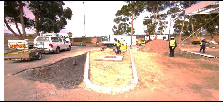
STORAGE TANKS INSTALLED AND TESTED, COMPACTED WITH RIVER SAND AND FITTED WITH TWO MANHOLES AND FOUR MONITORING HOLES
