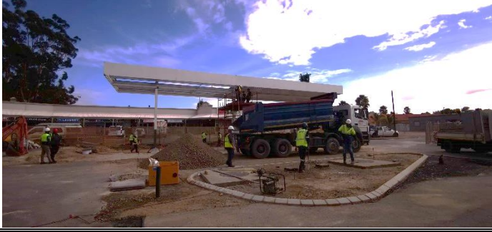
TWO FILLER PODS – FUEL TRUCKS WILL CONNECT DIRECTLY TO FILLER PODS TO REFILL STORAGE TANKS
