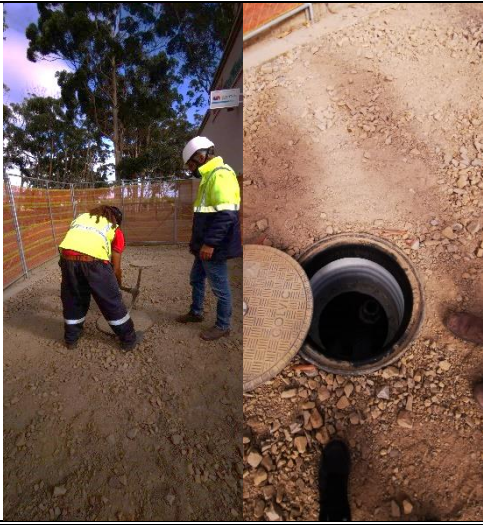
OIL SEPERATOR CHANNEL LEADING TO OIL SEPERATOR TANK
