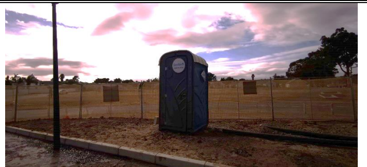
CHEMICAL TOILET SUFFICIENT FOR 15 WORKERS - ART WELDING TEAM
