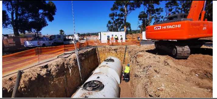
STORAGE TANKS COMPACTED AND TESTED – 24 FEBRUARY 2021
