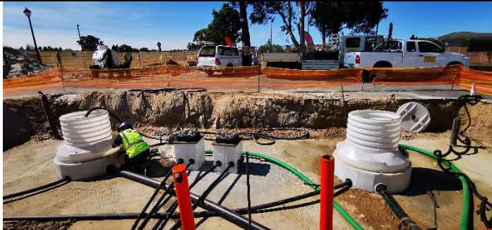
GREEN PIPES REPRESENTS SUCTION LINES FOR PETROL AND DIESEL FEED TO PUMPS
