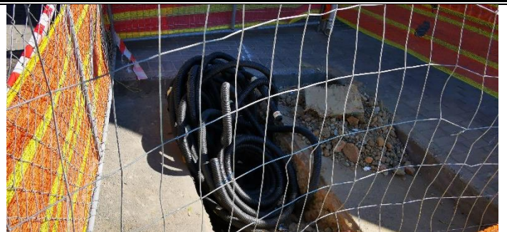
SLEEVES FOR ELECTRICAL CABLE LEADING TO DB BOX
