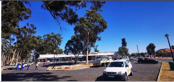
AVAILABLE PARKING AREA PRIOR TO CONSTRUCTION PHASE
