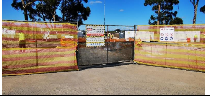
DRIVE IN ENTRANCE GATE TO CONSTRUCTION AREA
