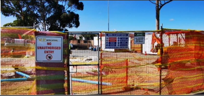
WALK IN ENTRANCE GATE TO CONSTRUCTION AREA
