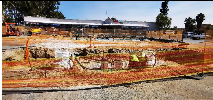
GREEN PIPES REPRESENTS SUCTION LINES FOR PETROL AND DIESEL FEED TO PUMPS
