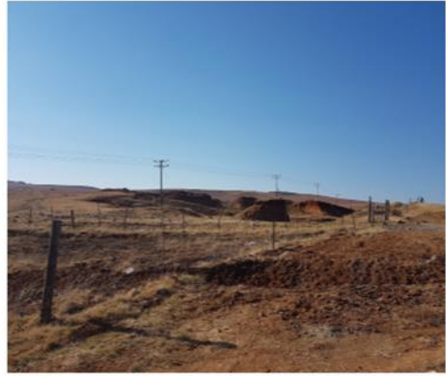
Excavations at site entrance next to R56
