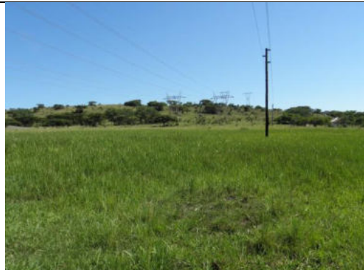
Photo 12: Power line traversing the HS (Pylon placed within the seasonally saturated zone).
