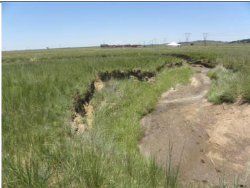
Photo 8: Portion of channel exposed to bank erosion
