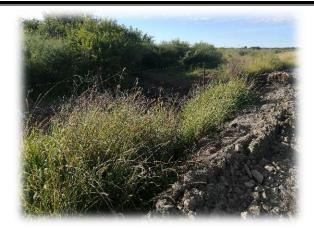
High velocity and volume flow during the previous weeks have resulted in some of the stabilizing material being washed away. This is mainly due to inapropriate culvert size
