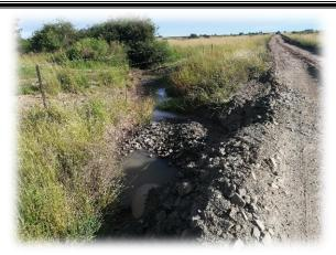
A larger culvert should be installed and the stabilizing matial reapplied following the rainy season.
