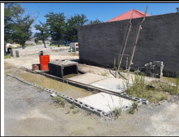
Wash bay that drains into an oil sump.
