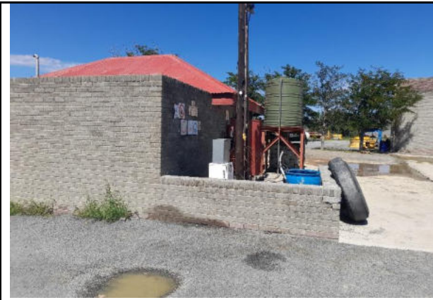
Diesel storage tank enclosed in a properly bunded area.
