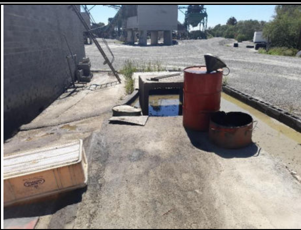
Wash bay that drains into an oil sump.
