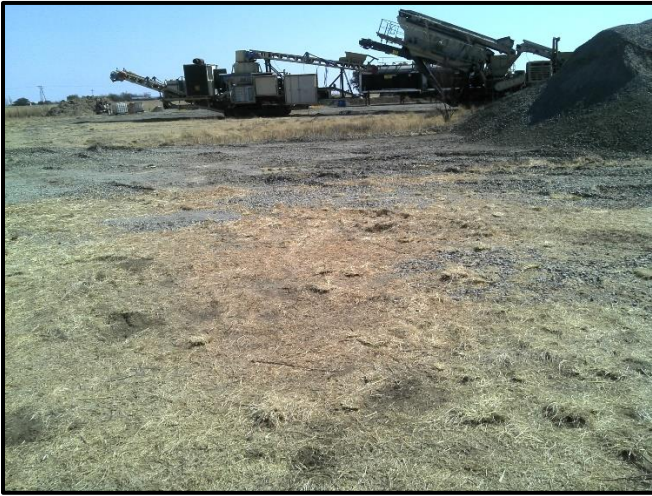
Figure 5. General Site conditions.
