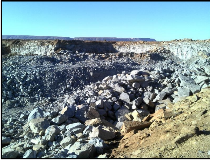
Figure 5. General Site conditions – existing quarry
