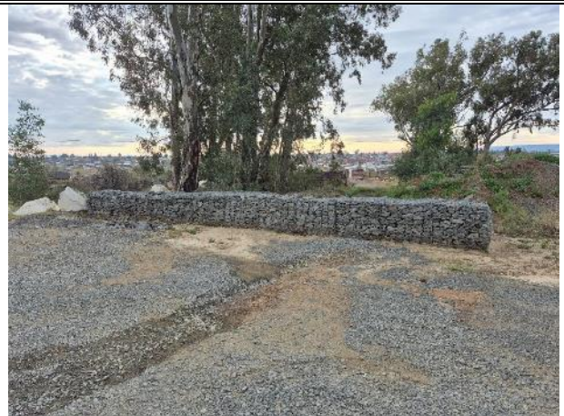
Gabion baskets added to control stormwater runoff
