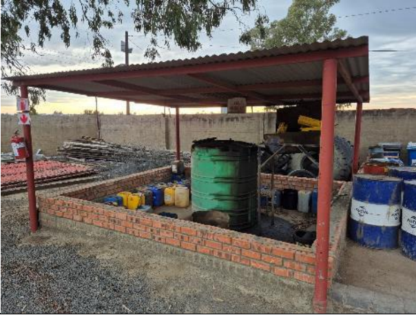
Hazardous materials storage area. Note bund added to the cement slab in the righthand picture
