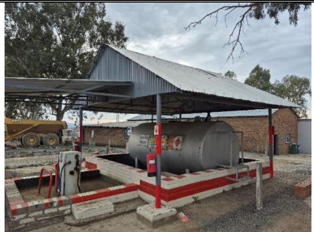
Diesel tank bunded area to be increased and sealed
