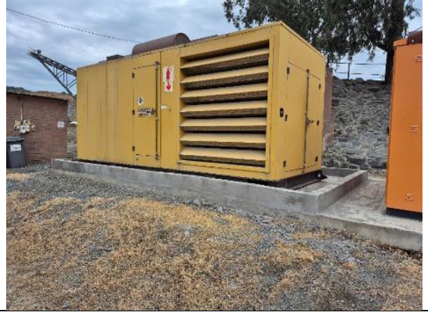
Generator fitted with a bund wall
