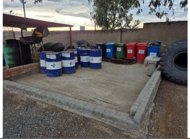
Hazardous materials storage area. Note bund added to the cement slab in the righthand picture
