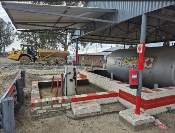
Diesel tank bunded area to be increased and sealed
